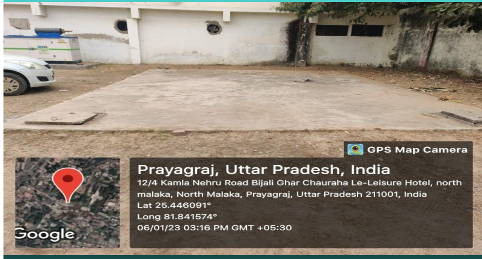
Rainwater Harvesting Chamber in Commerce Department
